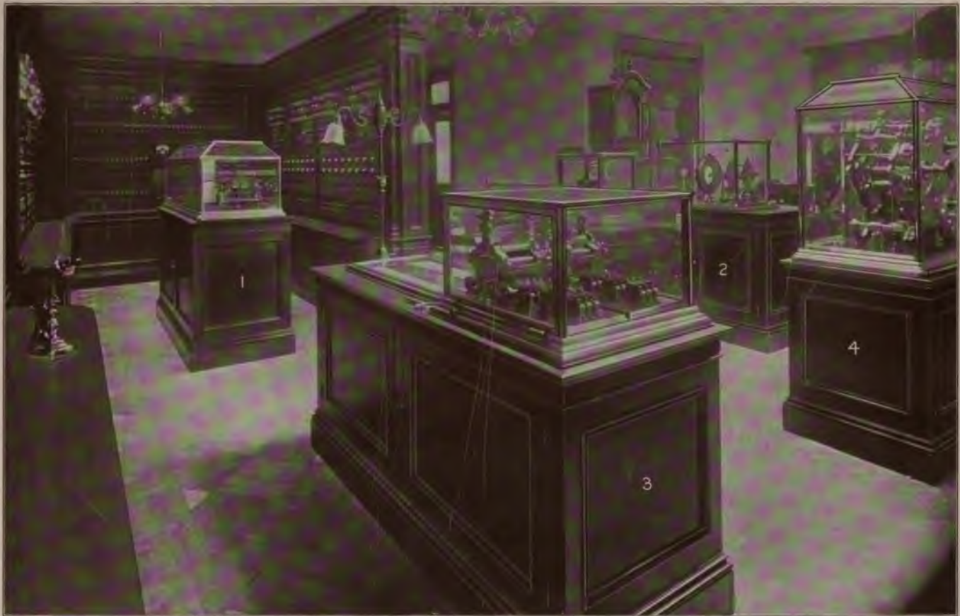
1, Automatic repeater; 2, automatic line tester; 3, multiple pen register; 4, manual dial transmitter.
